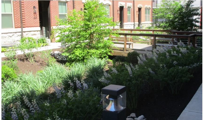
Installing a bioretention basin abutting existing impervious area can be an excellent Stormwater Management Banking and Trading strategy.
